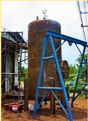
Air Receiver Tank Client: Cardinal Health Location:- Amata City Company:- USA
