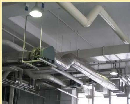
Exhaust Duct for Machine Client: Toyoda Gosei Amata Nakorn
