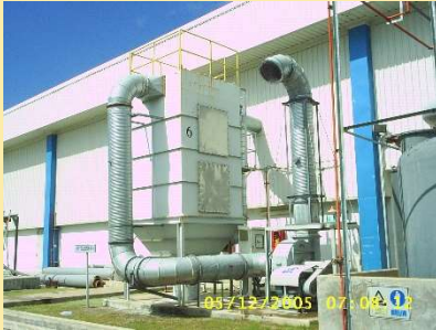
Dust Collector @Facility
