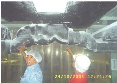
Ducting at Stripping
