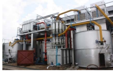
Supply and Install Mixing Tank Thai Paper Mill, 8 Million Baht
